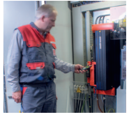
State-of-the-art frequency converter provides the power for the speed-controlled high-pressure pump drive
